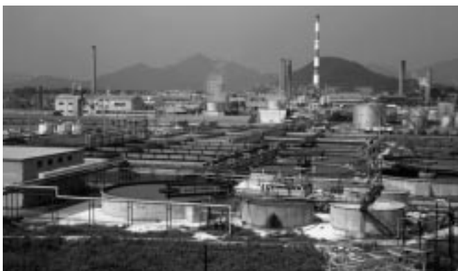
Wastewater treatment facilities at the Hofu Plant
