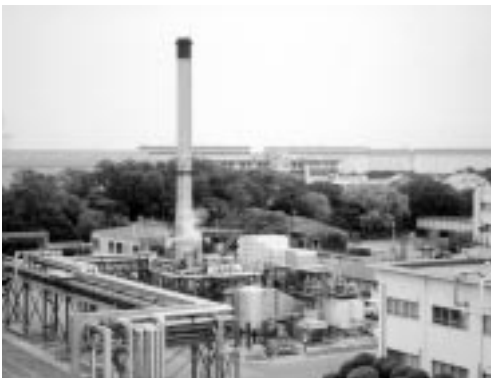
Cogeneration facilities at Kyowa Yuka's Chiba Plant
