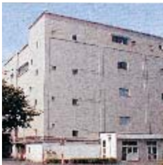
Building reinforcement for earthquake resistance
