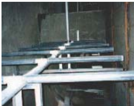
O 2 Magnum membrane tube diffusers (Shingashi Treatment Plant, Tokyo Waterworks)
