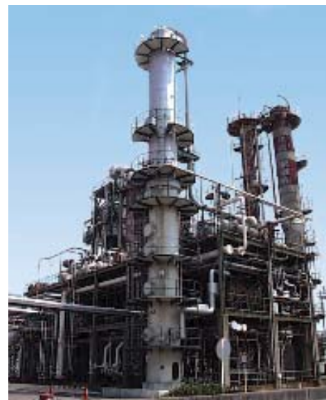
Energy-saving distillation column with vertical partitions
