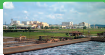
The BioKyowa Plant
