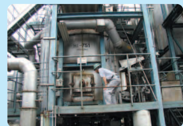
The decommissioned sludge incinerator
