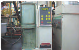
A solvent recovery system at the Pharmaceutical Research Institute
