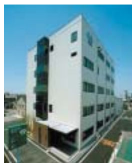
The quality management building at the Sakai Plant
