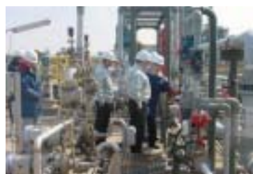
Chinese trainees study wastewater treatment facilities.
