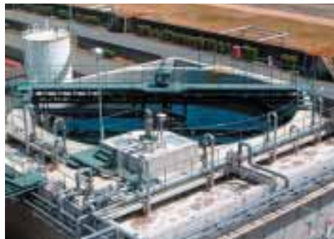
Yokkaichi Plant wastewater treatment facility expansion
