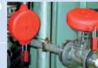
Valve lockout system
