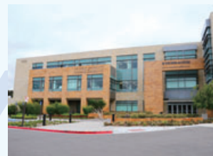
The facility where LIAI and KKC work together
