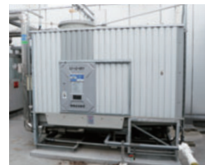
New closed cooling tower
